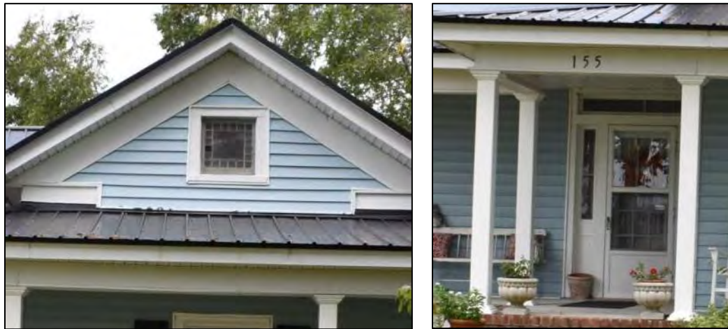
Figure 29: Left, detail of gable window; right, detail of front door
