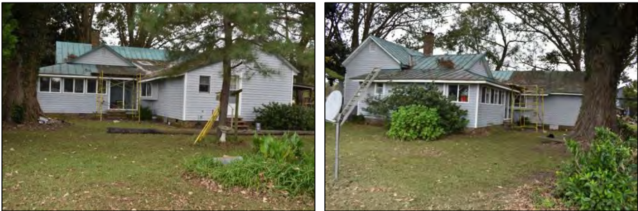
Figure 60: Left, east rear elevation; right, east rear and south side elevations
