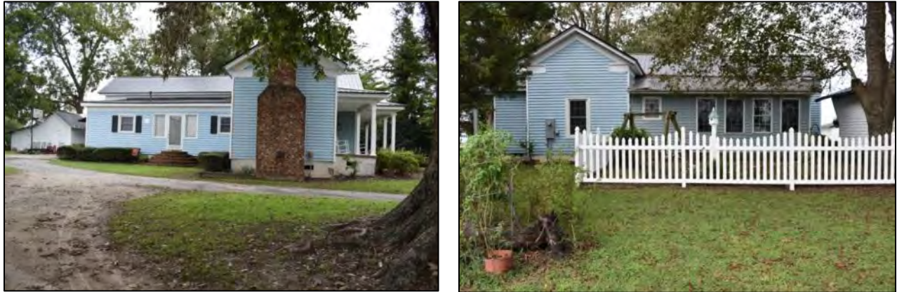
Figure 28: Left, western elevation; right; eastern elevation
