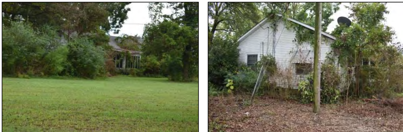
Figure 46: Left, view of house looking to southeast; right, northern elevation
