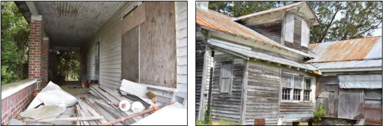
Figure 56: Interior view of porch, looking north; right, view of southern elevation
